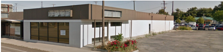
Current Building Before Renovation Project
